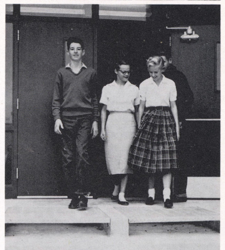
Stuart Brown, Marion High and Jan Durham inspect our new buildings.
